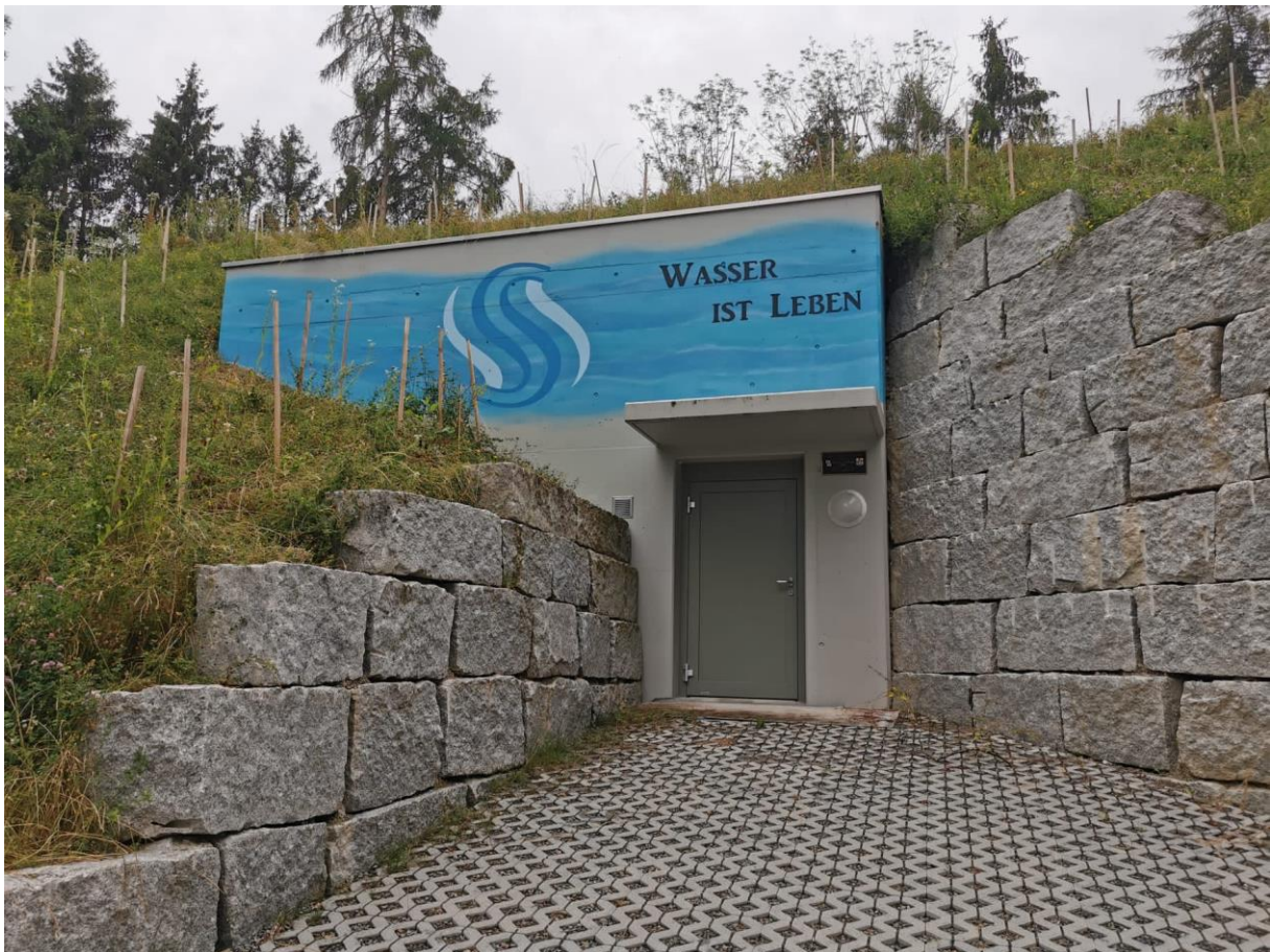
Foto: Reservoir Brandhalde, Sins (ts)
